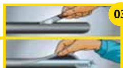
03 Longitudinal cutting of Izocamflex with a knife
